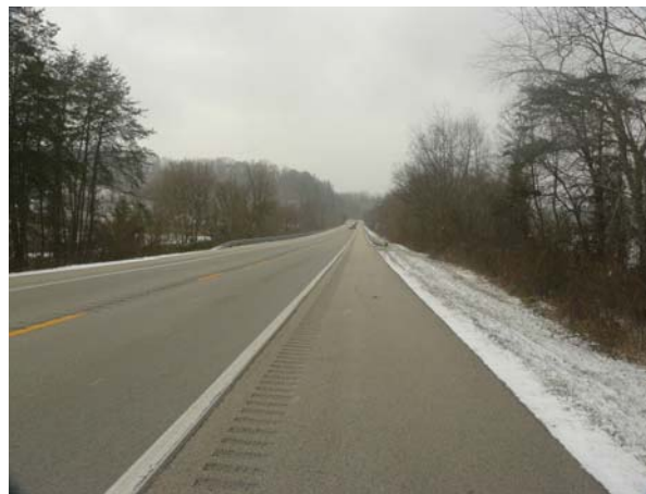
Photograph 1 –Looking Southeast Near Western End of Segment 1B
