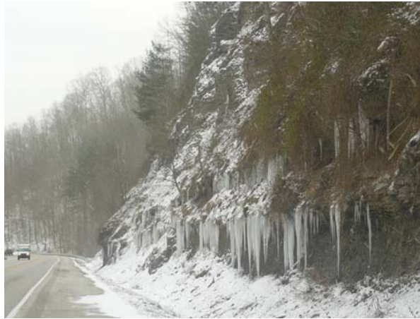
Photograph 2 – Rock Cut Slope along Southern Side of Segment 1B at Mile Marker 49
